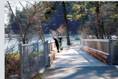
Footbridge east of Plantes Ferry Park
